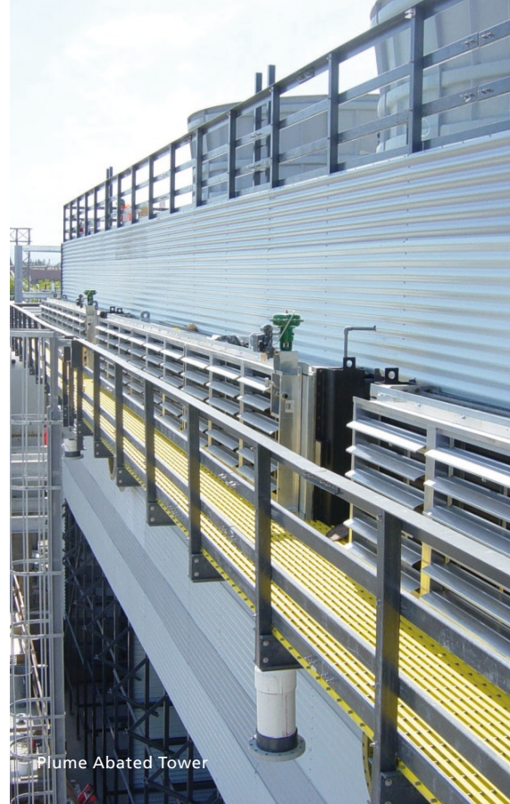
Vacuum Air Cooled Condenser
