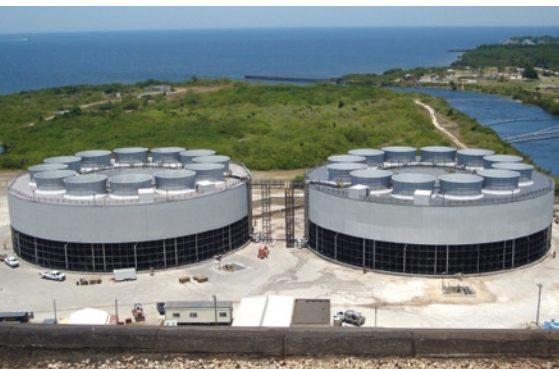
Florida, USA 2 x 12-cell counterflow, round fiberglass cooling towers
